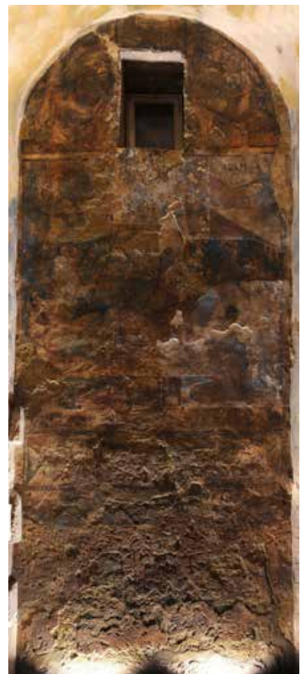
3.17. Raking light photo of South wall, West aisle, showing the plaster's spreading phases
