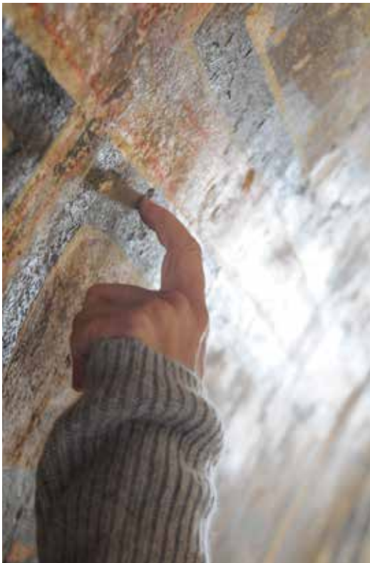
3.19. Layer of natural resin (shellac) applied at the time of the 1970's conservation
