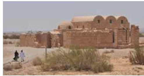
1.4. The main building at Qusayr ‘Amra
