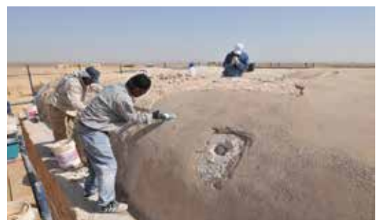
3.16. Application of layers of lime mortar on the vaults' extrados
