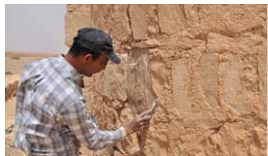
3.15. Final smoothing of mortar in repointed areas
