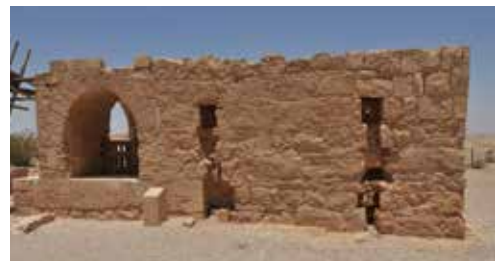
1.5. The saqiya annexed to the main building
