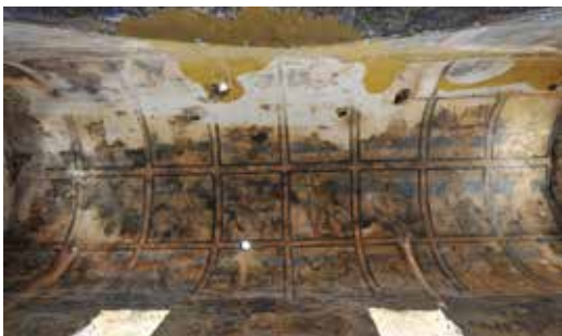
2.9. Aisle IC (east)
